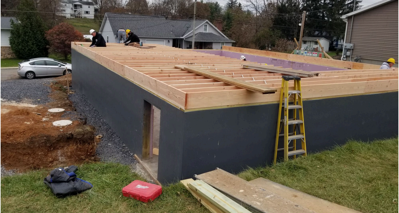
Home Foundations Being Constructed
