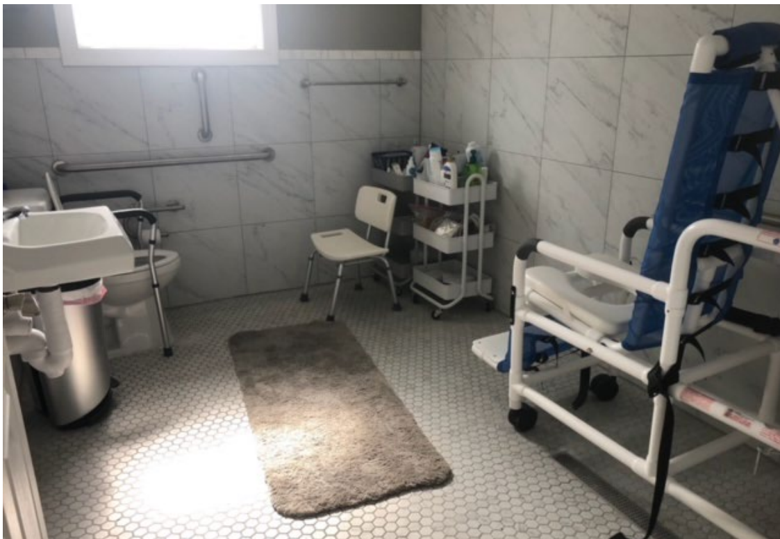
Bathroom After Renovation (Accessible Renovation and Equipment Allows Residents to Bathe and Use Toilet Independently)
