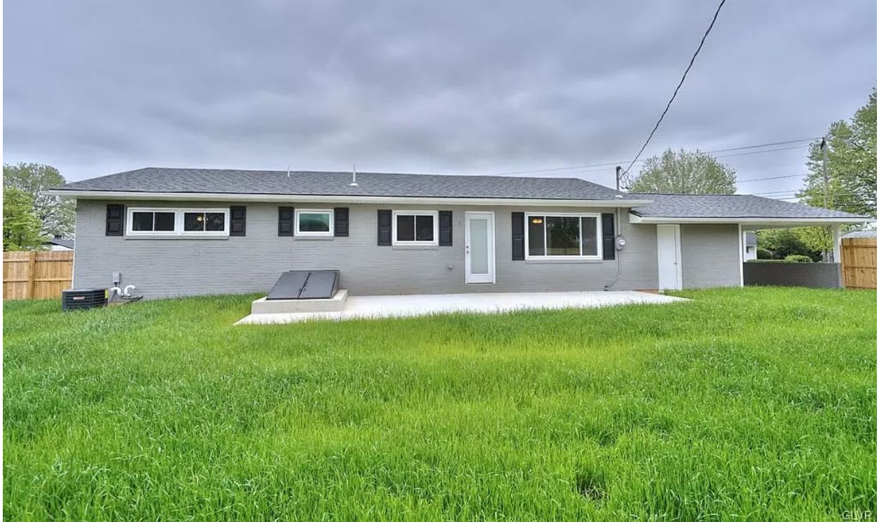
Before Accessibility Modifications (note: no ramp for a wheelchair user)
